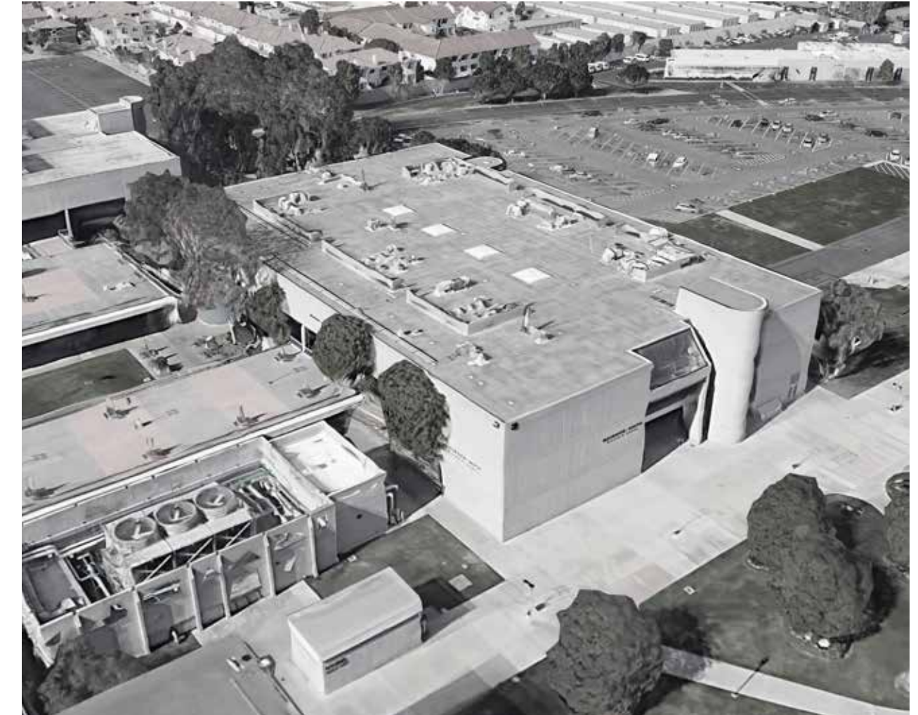
EXISTING SEM BUILDING SOUTH WEST CORNER
