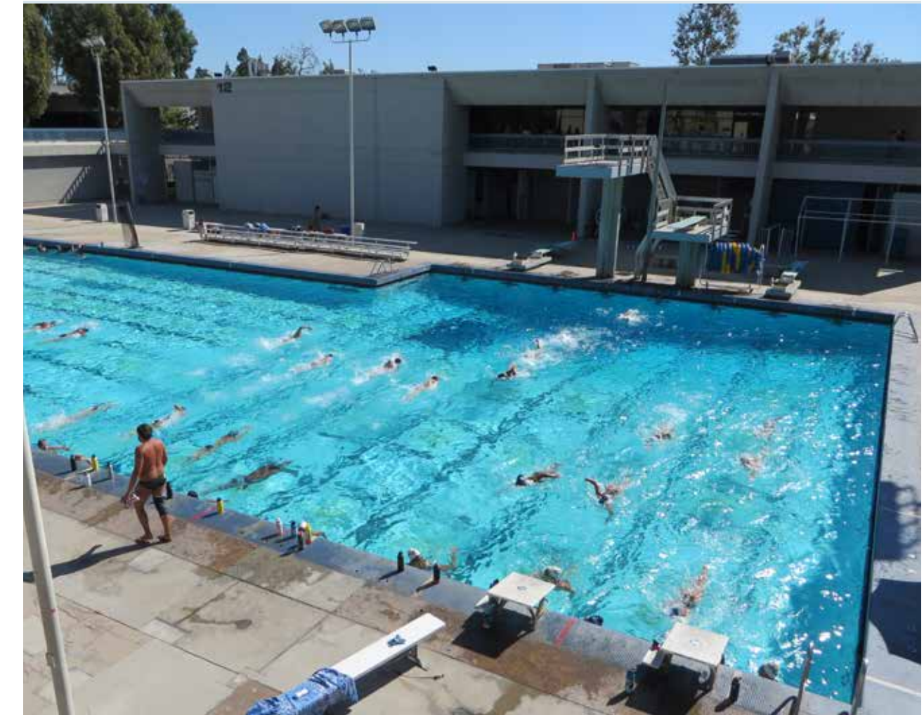
EXISTING SWIMMING POOL
